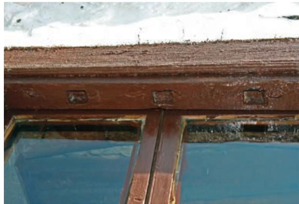
FIGURE 64 Detail of iron fasteners and rectangular holes on window frame, view from the exterior
