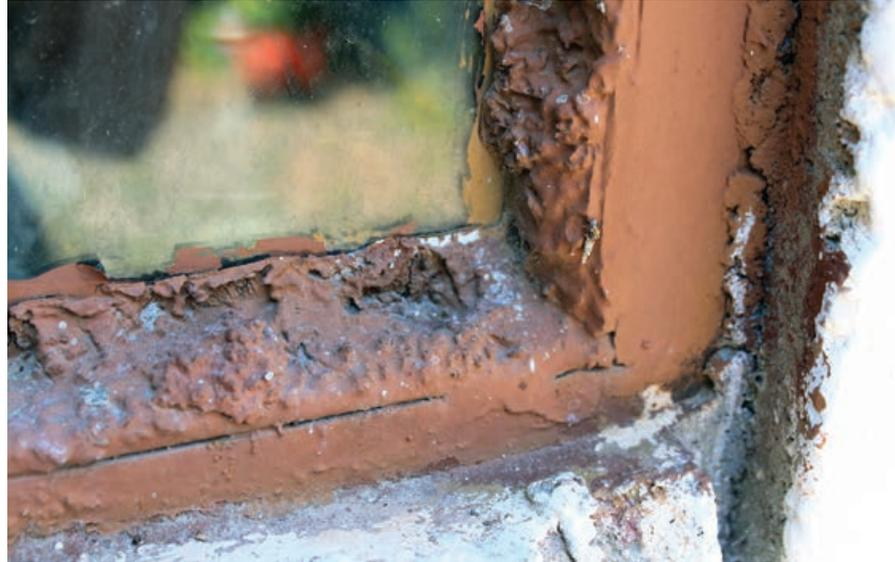
**FIGURE 54** Detail of plaster on sash
