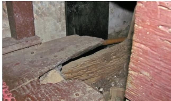
FIGURE 69 The concrete floor slab does not extend underneath the Bishop's throne
