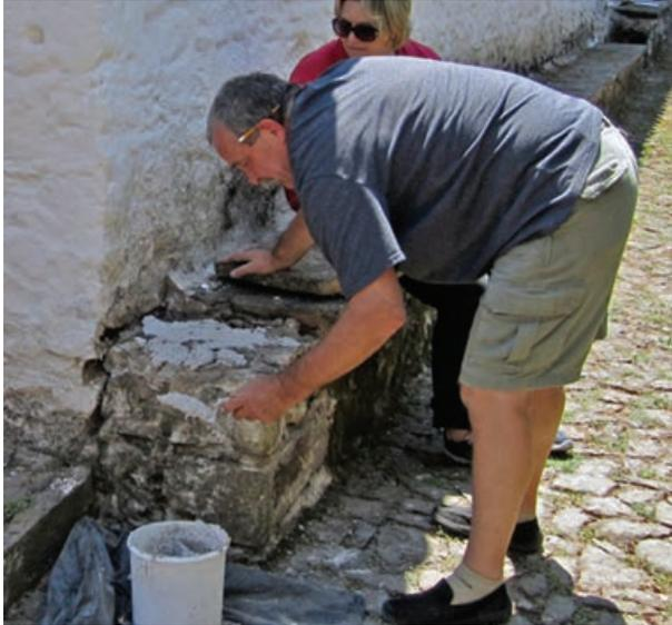
5. The mortar was hand-troweled onto the top of the bench.
