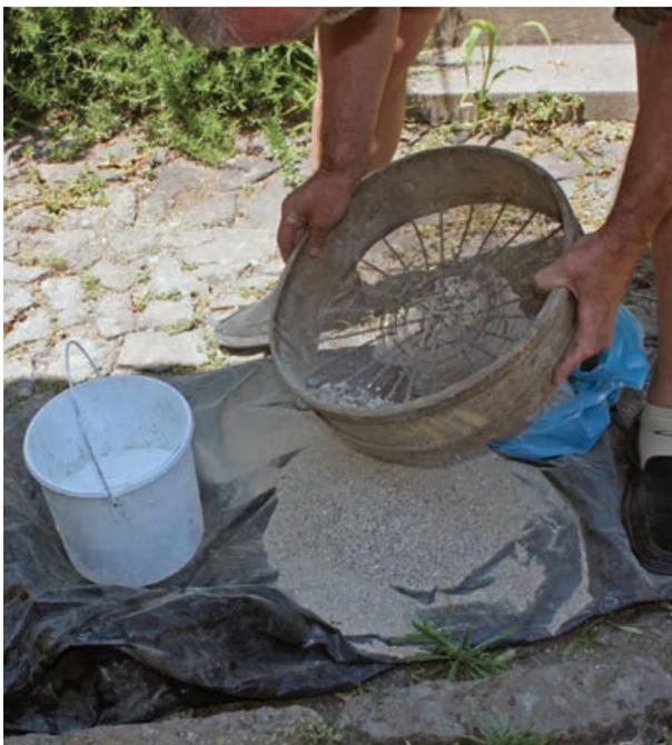
3. New pointing mortar was mixed, consisting of slaked lime putty, premixed and aged on-site, mason sand from a nearby supply yard, and potable water.
