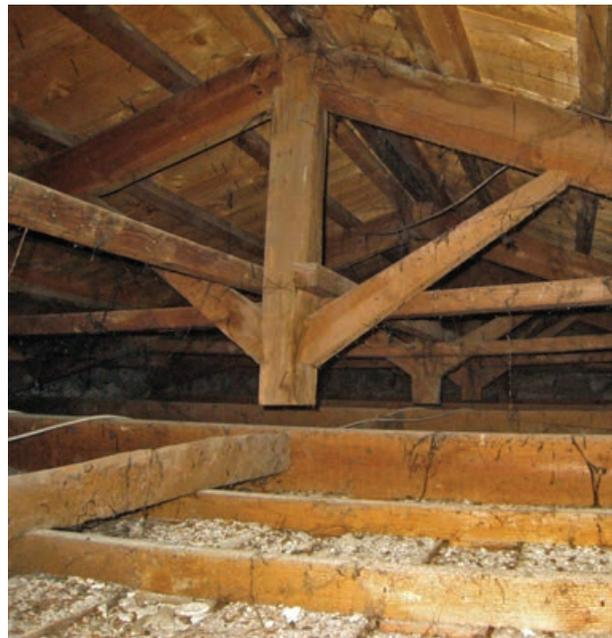
FIGURE 33 Main roof wood framing
