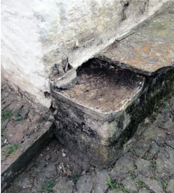
1. The cement cant at the rear of the seat was removed using hand tools and the bench seat was removed by hand.
