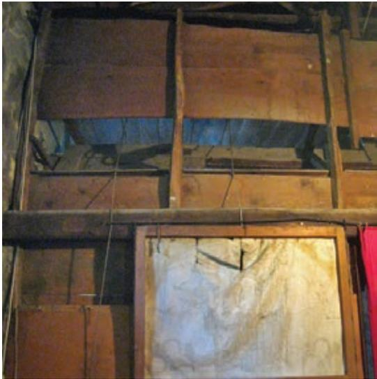
FIGURE 75 The rear of the iconostasis with unfinished framing members
