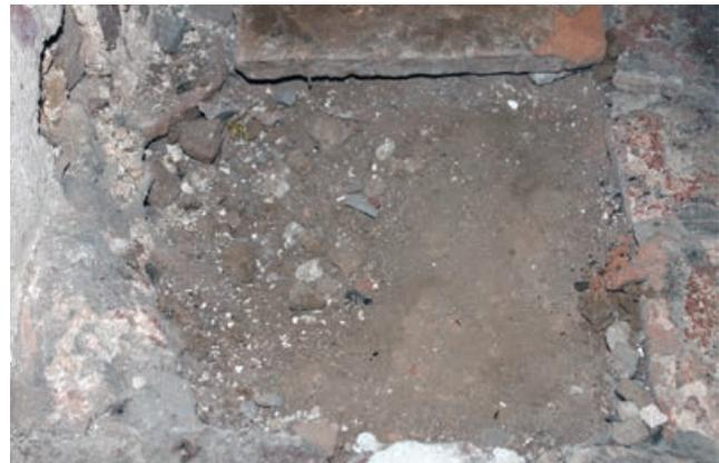
FIGURE 67 Floor tiles and soil substrate in the narthex
