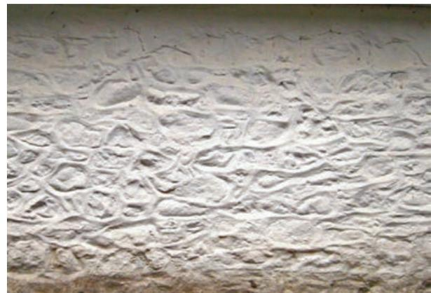
FIGURE 21 Local andesite stone was used for the walls of the Katholikon of Moni Perivolis
