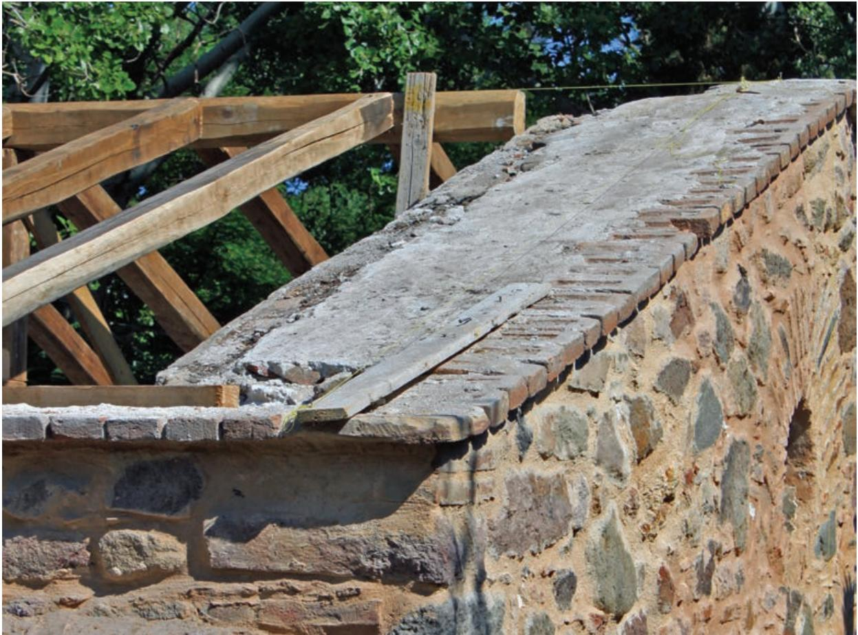
FIGURE I27 Soffit capping the top of the walls of the church
