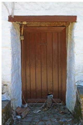
**FIGURE 40** Door D2, from the interior, showing wood battens
