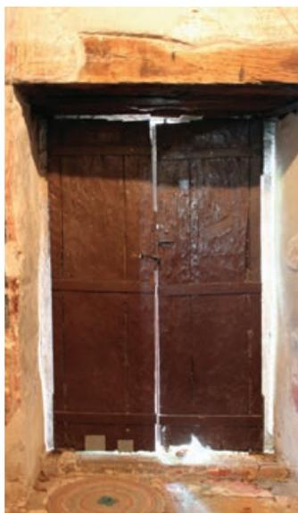
FIGURE 37 Door D1, from the interior, showing steel batten straps
