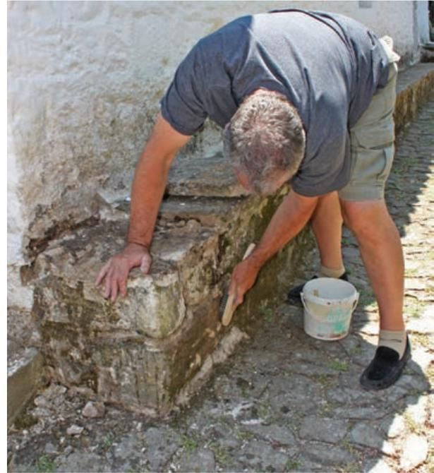
2. All hydraulic cement from the mortar joints on a portion of the North face and on the East end of the bench was removed by hand. All mortar joints were cleaned to expose the clay-and-sand setting mortar. The existing limewash finish was brushed to remove all biological growth (lichen) on the bench and on the adjacent façade wall. The entire mock-up area was rinsed lightly with fresh water.
